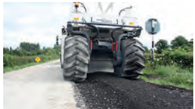
In situ pavement recycling with bitumen emulsion
